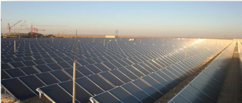
District Heating (and Cooling)
